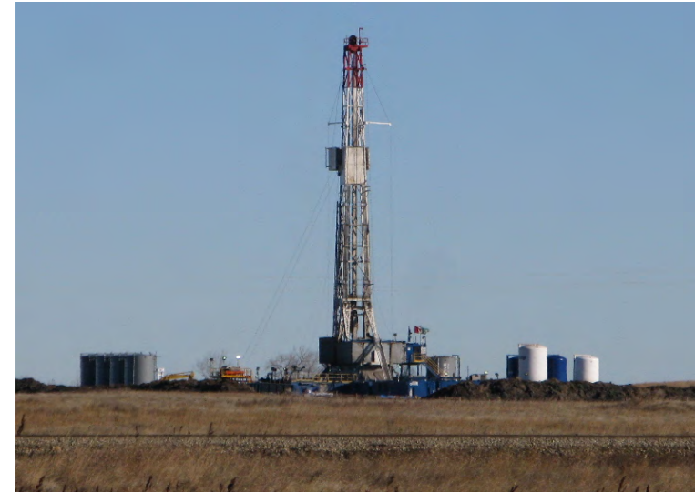
Injection-well 4B5-06-02-08W2M to the Winnipeg and Deadwood Formations at ~3350 m depth
